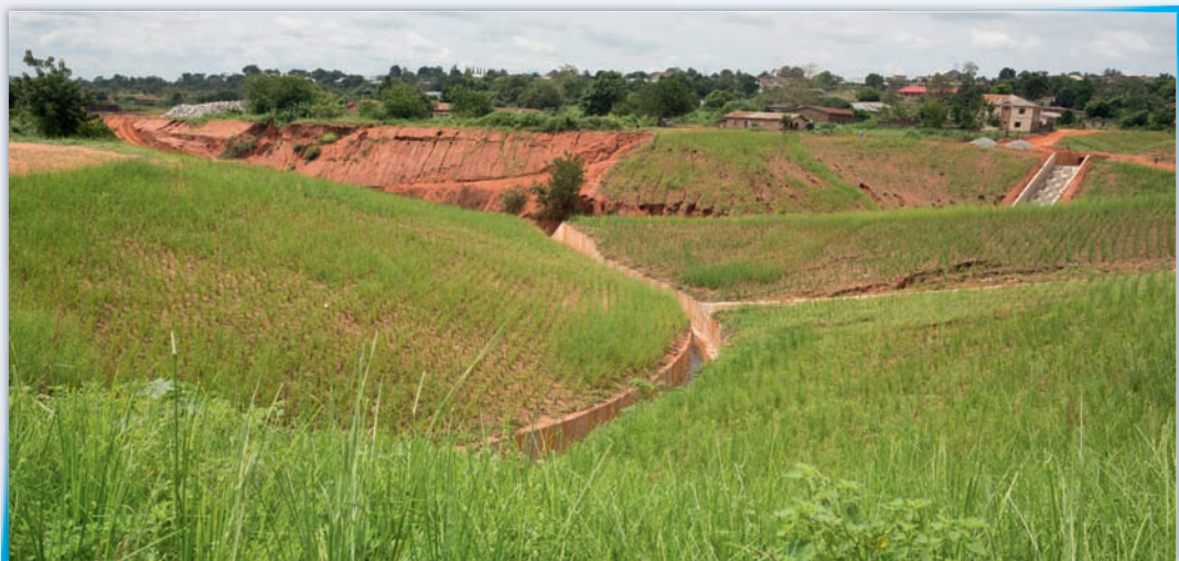
Anti-erosion, water and soil conservation structures, Nigeria
