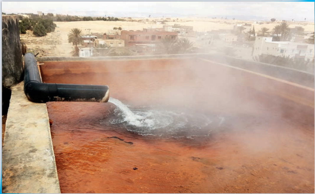
Hot water cooler in the old Kebili oasis, Tunisia
