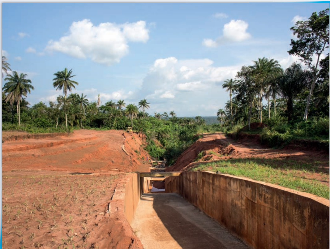
Rainwater drainage and anti-erosion infrastructures, Nigeria
